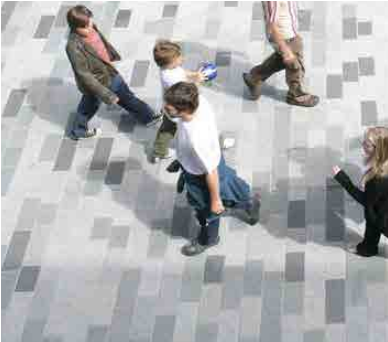
LANEWAY & PUBLIC GARDEN STONE UNIT PAVING (Stretcher bond perp. to path of travel)
