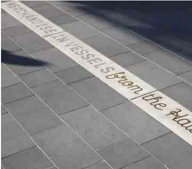
CONCRETE PAVING BANDS WITH BRASS INSERTS
